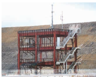
The Minamisanriku Town Disaster-Preparedness Policy Building will be governed by the prefectural government until 2031. The town is completely transformed as ground-raising work continues.
